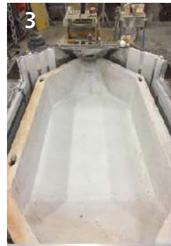
Figure 5: Installation of the liner into the steel shell
