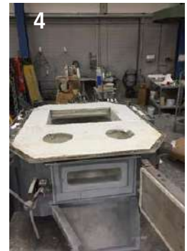
Figure 6: Installation of heating and roof blocks
